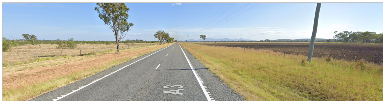
Figure 4.6 Burnett Highway Facing North
