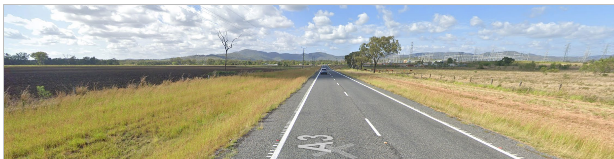
Figure 4.7 Burnett Highway Facing South
